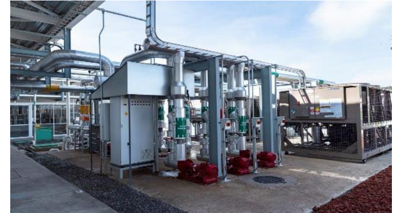
Water chiller system for OTC Plant
