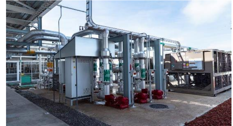
Water chiller system for OTC Plant
