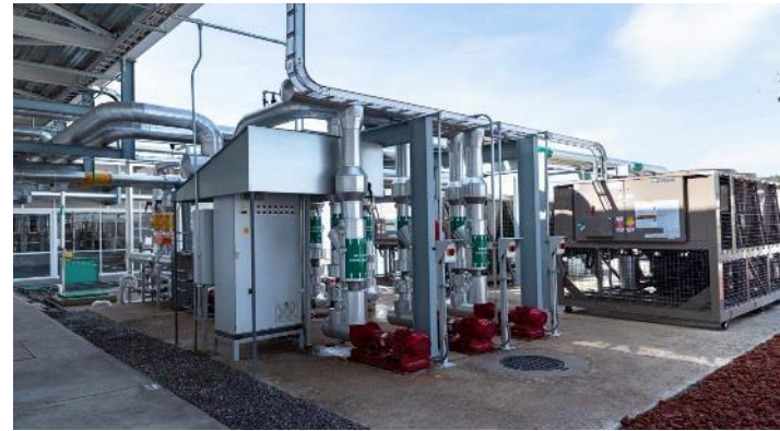
Water chiller system for OTC Plant
