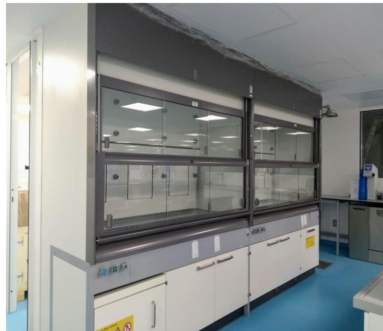
Quality Control Lab OTC Plant
