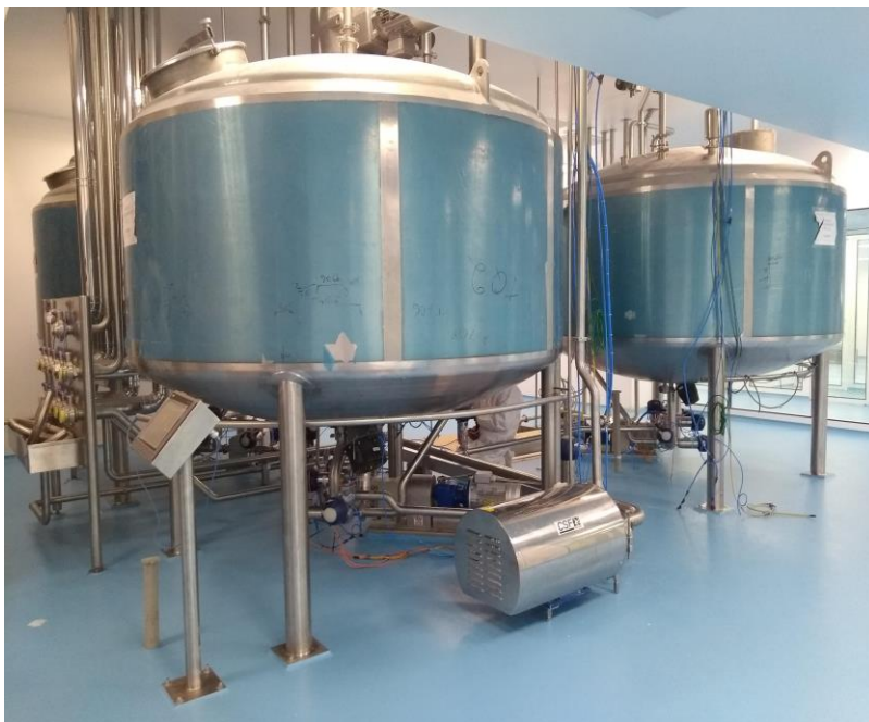
Equipment Installed OTC Plant Semi-Solids Production Line
