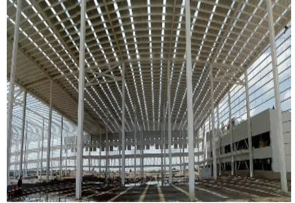
Progress on the Finished Product Warehouse (over 31,000 SQM)
