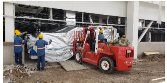
Manufacturing Equipment arrives at OTC Plant
